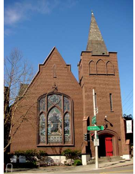
National Register #95001555 St. John's Presbyterian Church 25 Lake Street at Arguello Street Presidio Heights Built 1905
