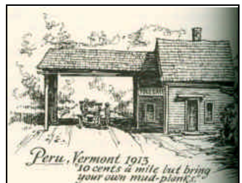
Entrance to an early Toll Road in Vermont. Sketch taken from the book: Eric Sloane's America
