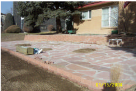
installing benches, etc.
