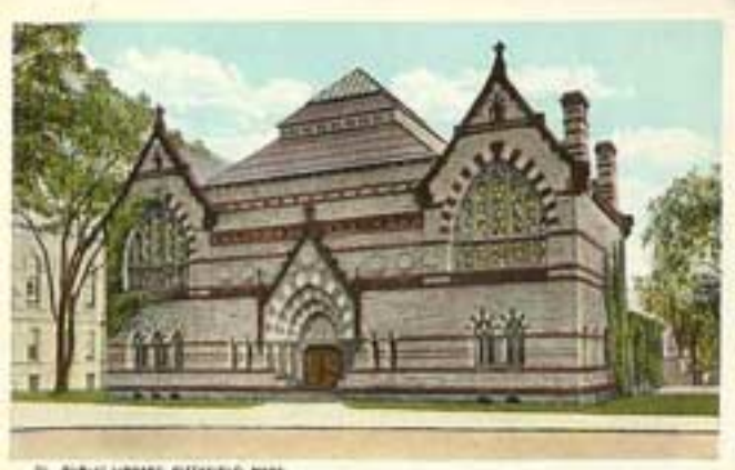
Pittsfield, Massachusetts Library built by the Dodge Construction Company
